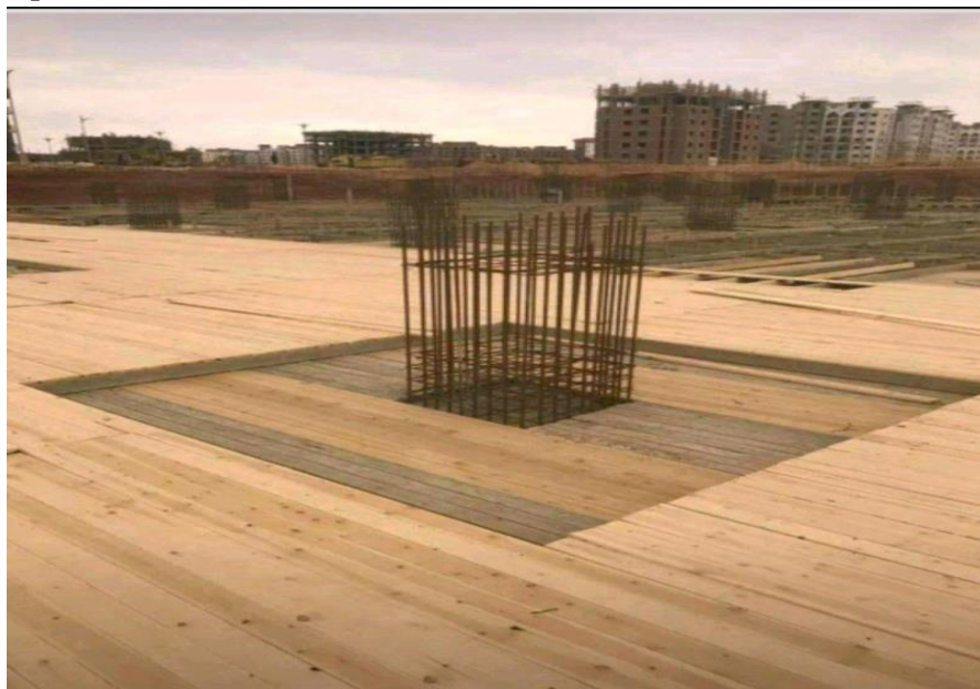
1) Site Preparation: Clean the site and prepare it for construction activities. Mark the locations for installing the drop panels according to the engineering design. 2) Installation of Drop Panels: Install the drop panels according to the engineered specifications. Ensure they are properly aligned and securely fixed in place.
